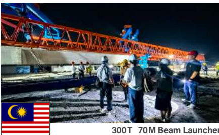
300T 70M Beam Launcher
