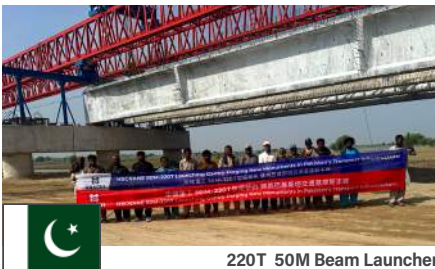
220T 50M Beam Launcher
