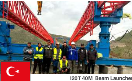
120T 40M Beam Launcher
